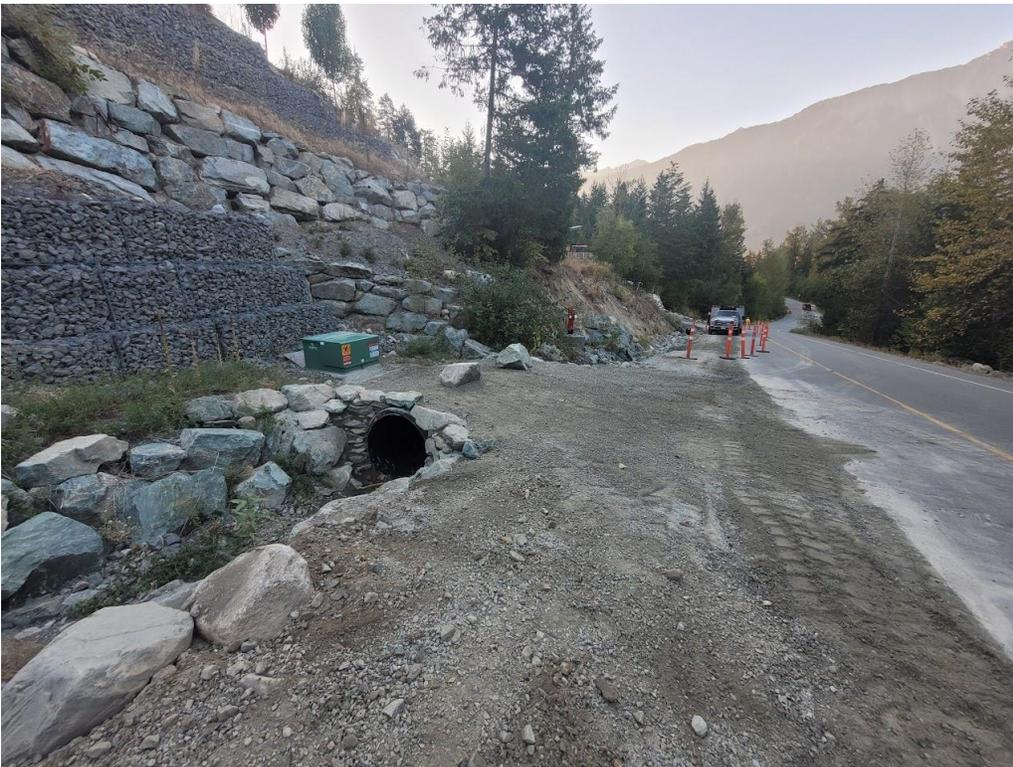
Figure 4 – Mackenzie Road washout repair
