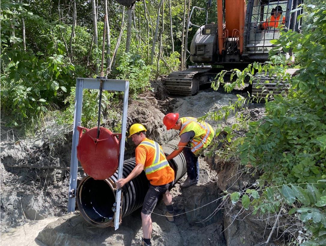
Figure 3 – One Mile Lake Inlet Channel culvert and gate valve replacement
