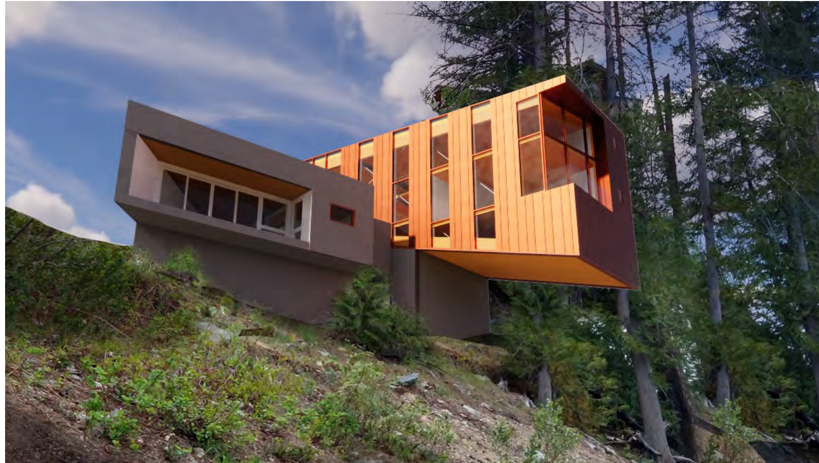
VIEW FROM DOWNHILL FROM EAST TO WEST
