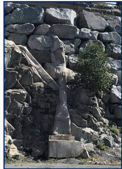
Visible utilities have a negative visual impact.
