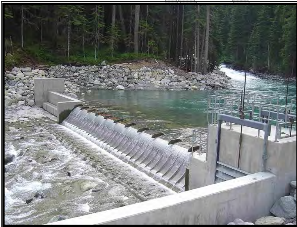
Run of River Power Inc.'s Brandywine Creek Hydro Coanda-type intake (photo from http://www.norrisscreen.com/products/hydroelectric.htm )
