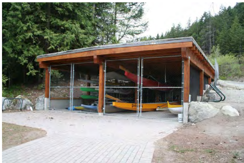
Secure boat storage facility with paved boat launch
