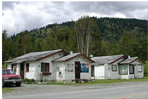
Mount Currie homes built of dovetailed logs
